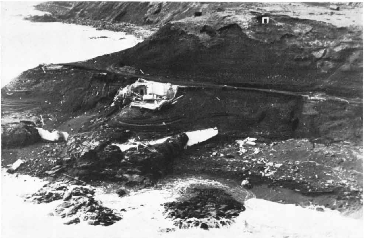
HUNDRED-FOOT "TIDAL WAVE," or tsunami, wrought impressive destruction at Scotch Cap, Alaska, in 1946. Reinforced concrete lighthouse that appears in top photograph was demolished, as shown in lower photograph, which was made from a higher angle.
